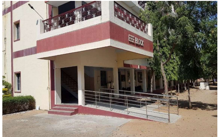
Ramp facility for EEE Department Block
