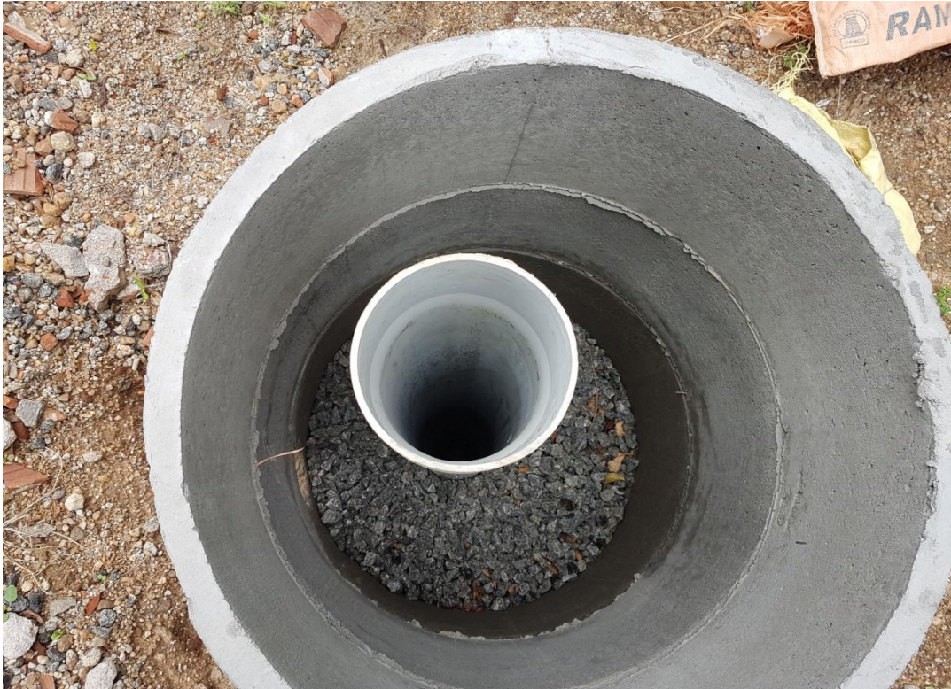
Plan View of Rain water harvesting pit
