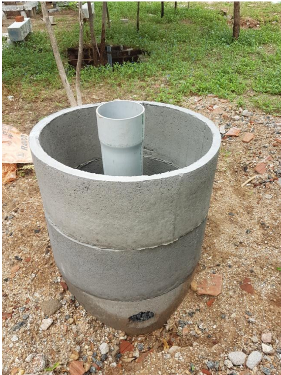
Process methodology – Percolation using medium sized gravel
