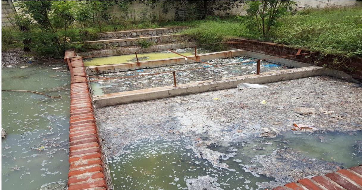
Sewage Treatment Plant of Capacity 50KLD
