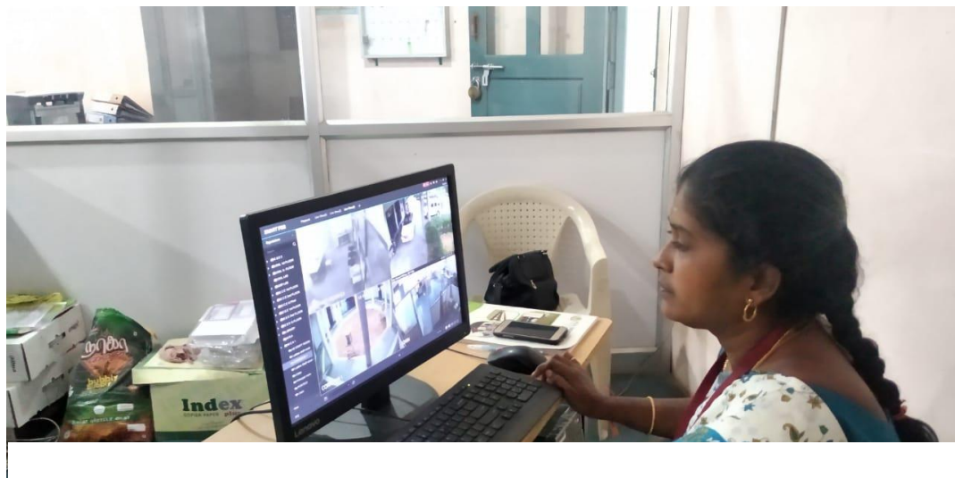
Fig: CCTV Monitoring Cabin
