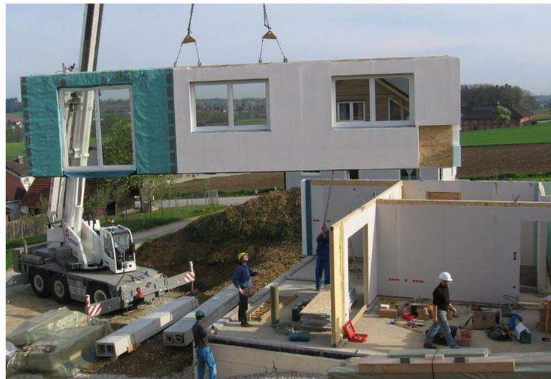
Prefabricated house construction
