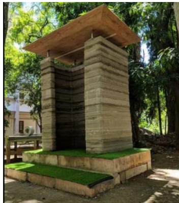
A 3D-printed building made using the newly developed technology. Image courtesy: IIT Madras
