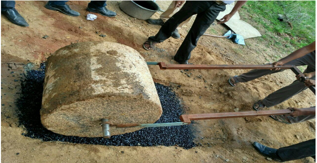
Demonstration on Composite Flexible Pavement Using Waste Plastics and Tyres
